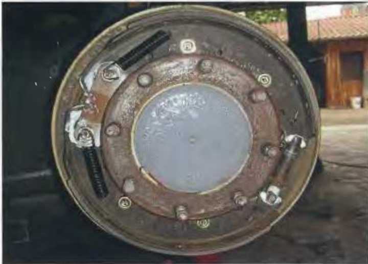
Before fastening the brake drums the new lined brake shoe was fitted.
